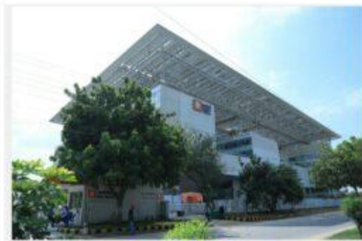
REC Limited HQ building
